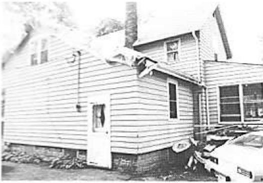
Wind & Storm Damage
